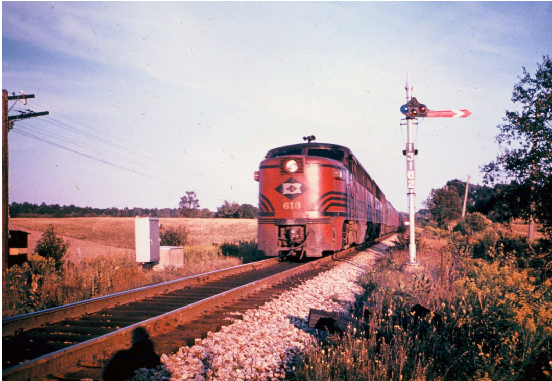
#10 “Black Diamond” northbound along Falls Rd., late summer 1958?
