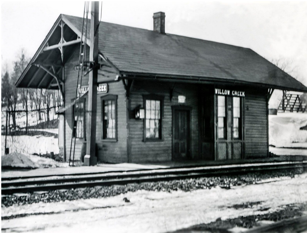
Willow Creek station, looking W
